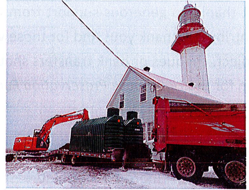
Installation of new septic systems (Photo : Ladd Johnson)
